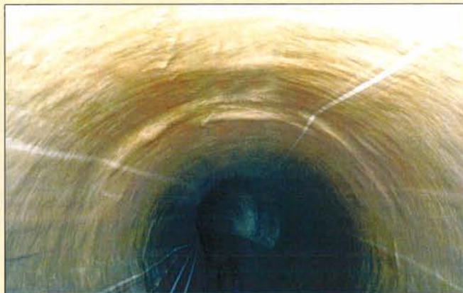
The newly-lined pipe is structurally improved, smoother, seamless and leak-free.
