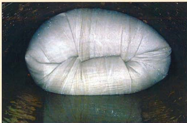
Pressure inverts the resin-impregnated felt tube through the host pipe.
