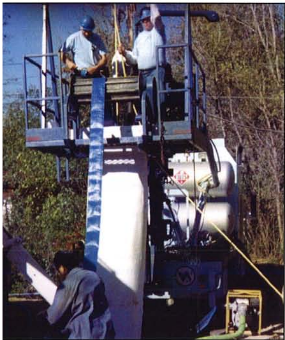
The inversion process, accomplished with a head of water, is relatively simple. On this project, inversion lengths ranged from 20 to 600 linear feet.
