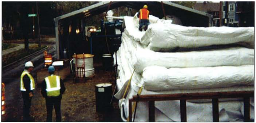
Above: Layers of felt are being examined as the crew prepares to inject the thermal-sensitive resin and catalyst system. Below: The resin-injected liner is lowered 75-feet to the sewer.
