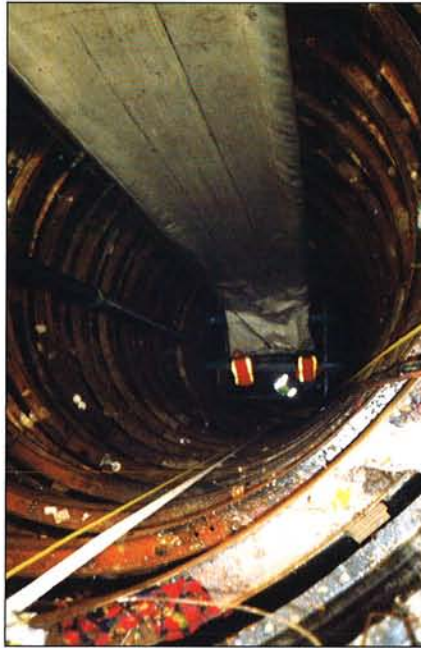
Above: Layers of felt are being examined as the crew prepares to inject the thermal-sensitive resin and catalyst system. Below: The resin-injected liner is lowered 75-feet to the sewer.
